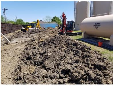
WATER UPDATE Hydro Resources, has finished the pilot hole and have almost completed the reaming operation to enlarge the hole to its full 16 inch diameter. Hydrologists are analyzing the core samples to determine the design parameters for the screen and gravel pack that go on the bottom. We are proceeding on schedule for a June completion date.
